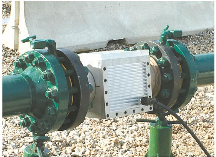
**Remote energy generation without fuel costs, without running wires across the miles and with little maintenance? Yes, with Lightning Master's In-Pipe Turbine Generator. Call 800-749-6800 to put this power to work for you.**
